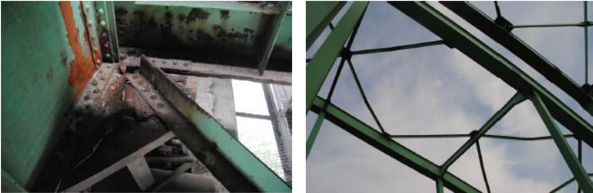
Figure 3. Disconnection and buckling of braces. Tennoh Bridge. Japan (Kawashima K (2012))
