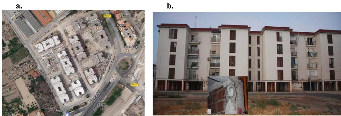
Figure 1. a) An aerial view of the San Fernando Neighbourhood (Source: Google Maps, 2017); b) Front façade of the surveyed building as damaged after the Lorca (Spain) 2011 earthquake and detail of a first floor damaged column. (Source: the authors).
