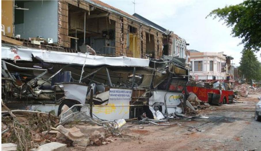
Figure 6. Example of out-of-plane wall failure from Christchurch earthquake (Fairfax, 2011).
