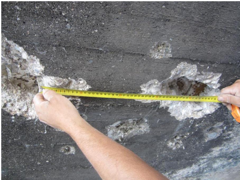
Figure 5. Distance between rigid reinforcement sets (author's photo)
