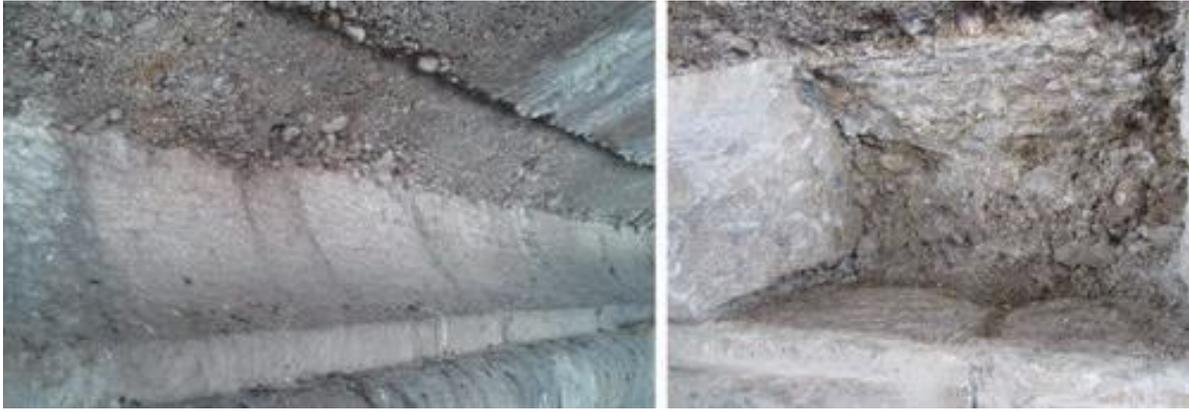
Figure 4. Abutment stone blocks at the left bank of the river and situation after their removal (author's photo)
