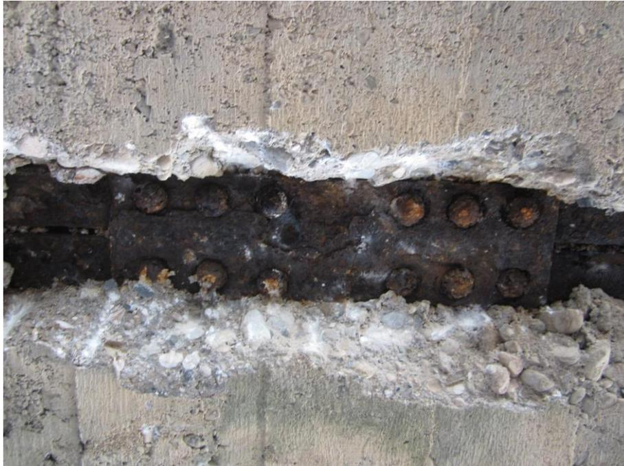
Figure 6. Connection of the rigid reinforcement (author's photo)
