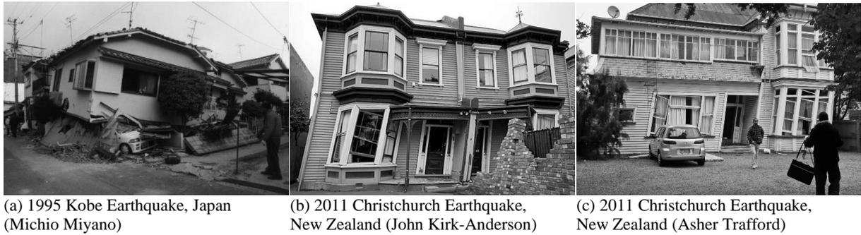
Figure 9. Examples of damaged 2-story houses. Considerable damage is concentrated in their first stories.
