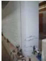
Damage of column at drift 1/100
