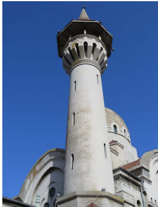
Figure 4. The minaret of "Carol I" Royal Mosque in Constanța (2017 photo)
