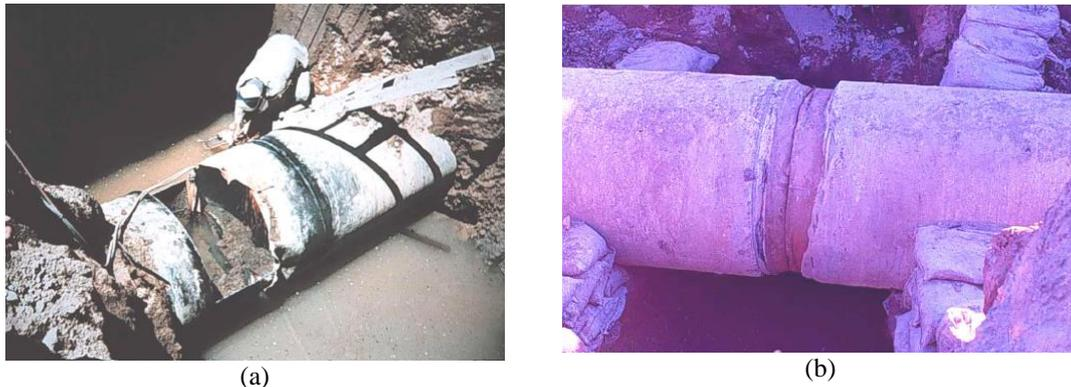
Figure 1. Failure of pipelines in Mexico City earthquake (1985): (a) fracture steel pipe and (b) concrete pipeline connection Failure (Berrones and Liu 2003)
